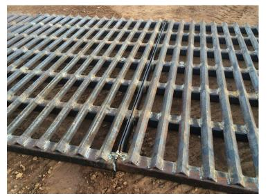
Rattle Grates are used for stabilized construction entrances. Rattle Grate provides the most effective method to reduce jobsite dirt and debris from being tracked onto public roadways.
